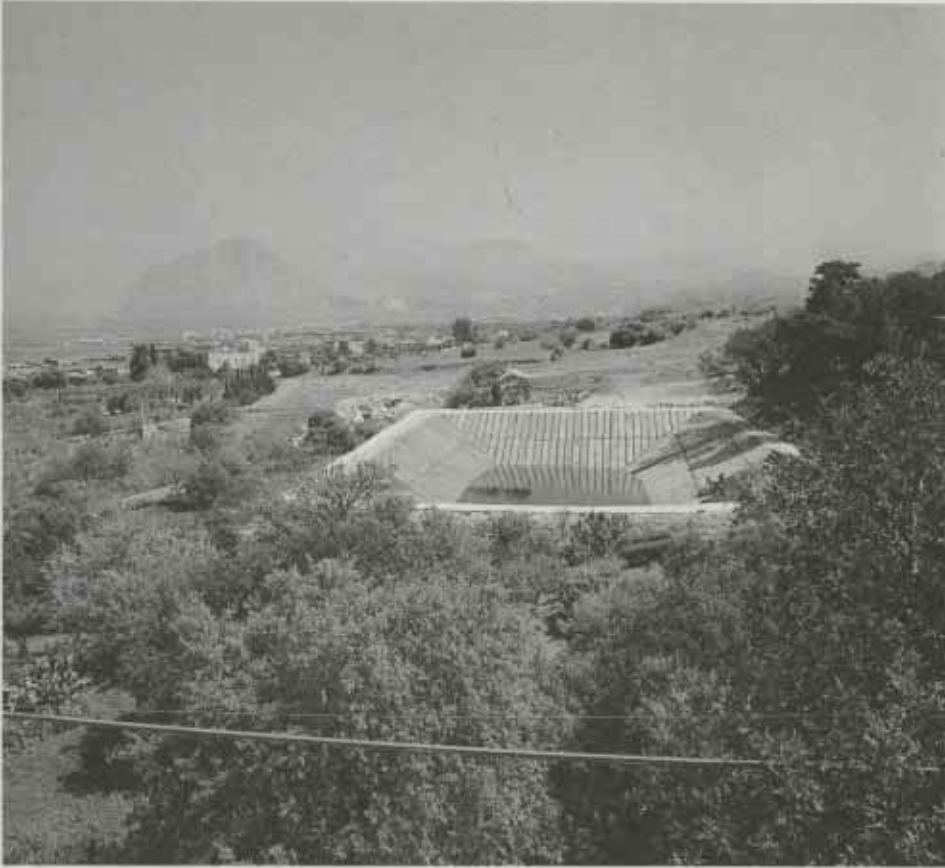
Earth based water reservoir. Finished work.
