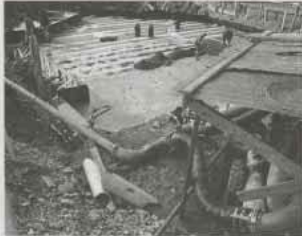
Detail of the pumping phase to lower the water level.
