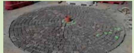
2017 - Roundabout in stone cubes (VR)
