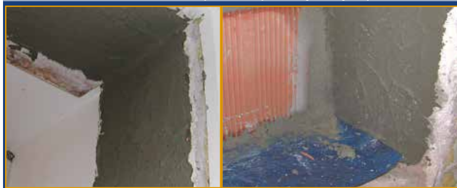
FONOPLAST, used as a separating layer, guarantees a damping level of "impact noise" of shared parts of buildings: shared staircases and corridors in apartment blocks etc.
