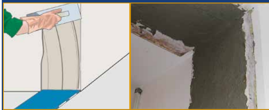
FONOELAST MONO, used on stairs as a separating layer, guarantees a damping level of "impact noise" of shared parts of buildings
