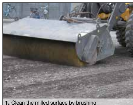
1. Clean the milled surface by brushing
