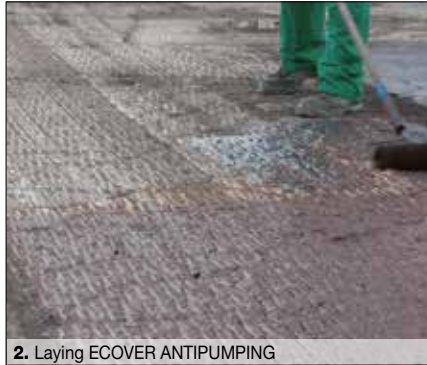
2. Laying ECOVER ANTIPUMPING
