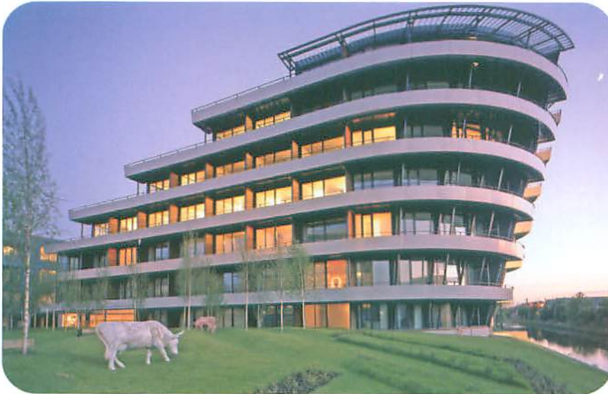
Large slabbed underground car park serving 125 luxury apartments at the Budenberg HAUS Projekte, Altrincham Manchester
