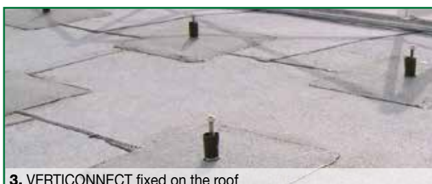
3. VERTICONNECT fixed on the roof
