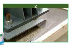
**BETON FLUID RAPID** must be mixed with clean water while maintaining a water/cement ratio lower than 0.40. The mix must be carried out by adding powder to the filler already wet with water (1).
