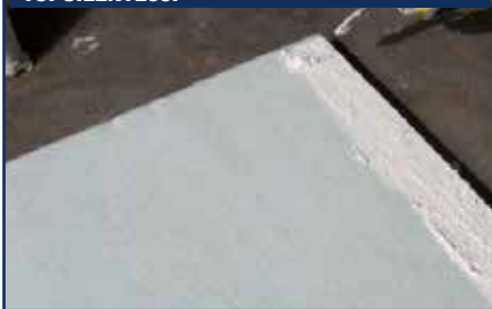
2. Spread with a spatula on the wool of TOPSILENTEco.
