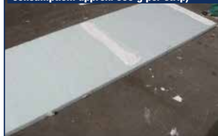
3. Apply two strips per panel (GIPSCOLL consumption: approx. 600 g per strip)
