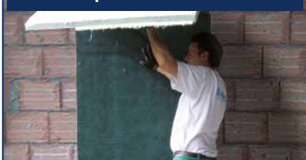
4. Place the panel on the wall.
