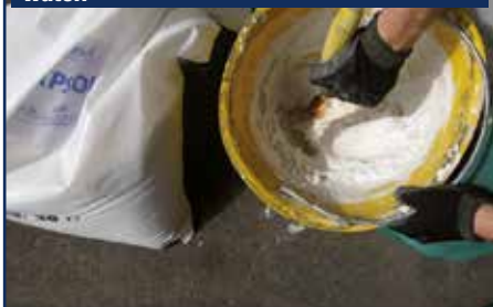
1. Mix the powder glue GIPSCOLL with water.
