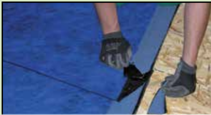
1. Smooth-off the corner of the upper edge of the overlap
