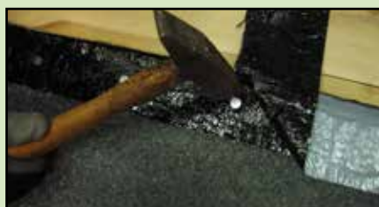
5. Nail down below the side overlaps
