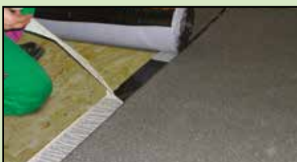
4. Remove the double-sided silicone-coated film protecting the adhesive selvage below
