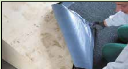
1. Remove the silicone-coated film
