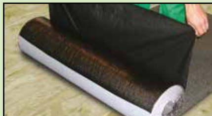
2. Peel off the silicone-coated film
