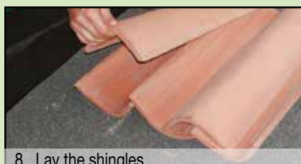
8. Lay the shingles
