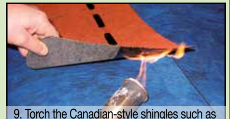
9. Torch the Canadian-style shingles such as COVERTILE on the Texflamina finish
