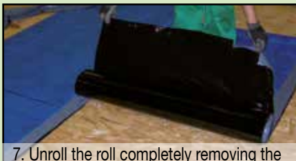
7. Unroll the roll completely removing the bottom film
