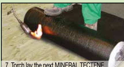
7. Torch lay the next MINERAL TECTENE TEGOLA EP membrane
