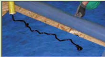
2. Extrude the HEADCOLL adhesive in the overlap area
