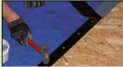
5. Nail the selvage of the sheets previously bonded
