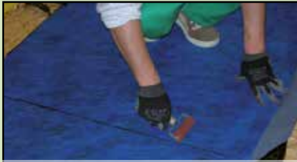
4. Carefully press the overlap area
