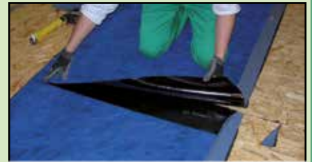
3. Place the upper edge on the adhesive spread
