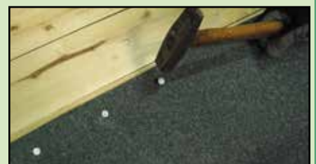
6. Nail down below the head overlaps
