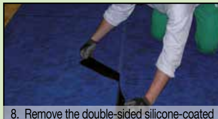
8. Remove the double-sided silicone-coated film protecting the adhesive selvage below
