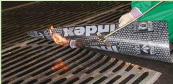
Flame-laying of the lateral and end-to-end overlaps so as to ensure perfect sealing against the passage of vapour
