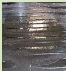
As torching continues, the heat-adhesive strips will assume a semi-liquid, glossy consistency: **the surface is now ready to receive the panels or rolls of insulation.**
