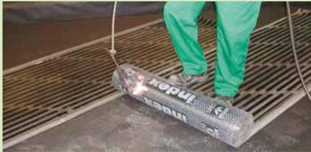
Flame-laying of the lower face of TECTENE BV STRIP EP
