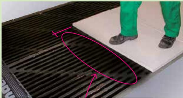
The insulation panels laid on the surface just torched must be bonded to the TECTENE BV STRIP EP by the pressure of the operator simply treading on them (this must be done over the entire surface of the panel).
