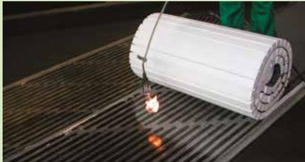
The THERMOBASE rolls which are unrolled on the surface just torched must be bonded to the TECTENE BV STRIP EP by pressure over the whole surface of the roll, exerted by the operator simply treading on them (this must be done over the entire surface of the panel or roll).
