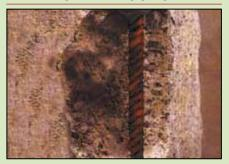
The formation of rust on concrete reinforcement bars caused by a number of factors lead to detachments and cracking. Bars protruding from concrete are exposed to rapid corrosion, which causes the concrete to deteriorate quickly, thus compromising the stability of the building work.
