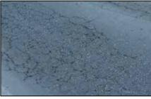
Through the cracks in the road paving, due to the "pumping" generated by the road traffic, rain water transports to the surface the fine parts of the layers not bound to be substrate, thus causing the progressive collapse of the road paving.
