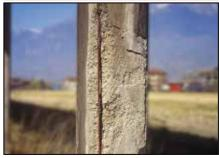
Some concrete repair work requires the application of considerable thicknesses without using formwork. Repairs to corners of beams or pillars, front cornices and wall-floor joining mouldings, requires the use of highly thixotropic mortar, with compensated shrinkage in order to avoid cracks and shrinkage hairlines.
