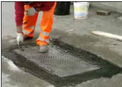
Create patches on concrete or industrial road or airport surfaces in a short time with a quick setting and easy to use mortar. Manhole cover fixing.
