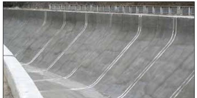
Hydroelectric channels, spray application
