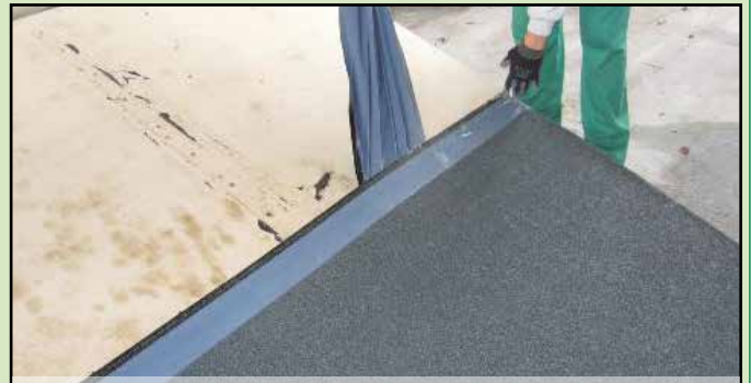
2. Apply the self-adhesive membrane
