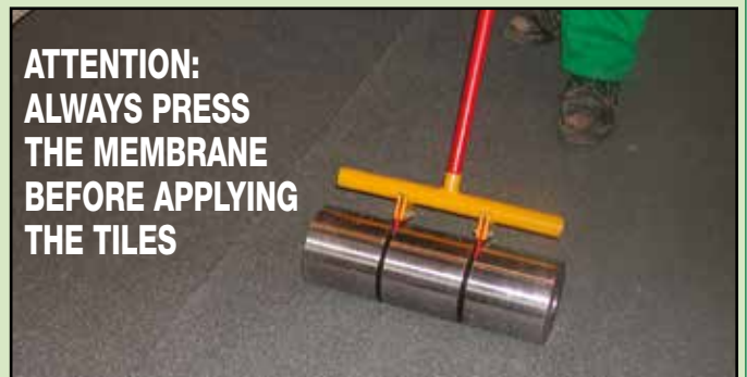
8. Press the whole before applying the tiles
