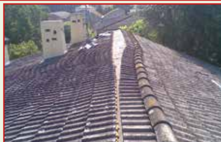
8. Press the whole before applying the tiles
