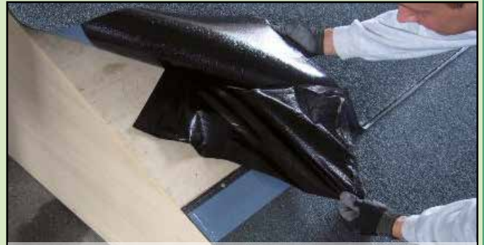
4. Apply the following membrane
