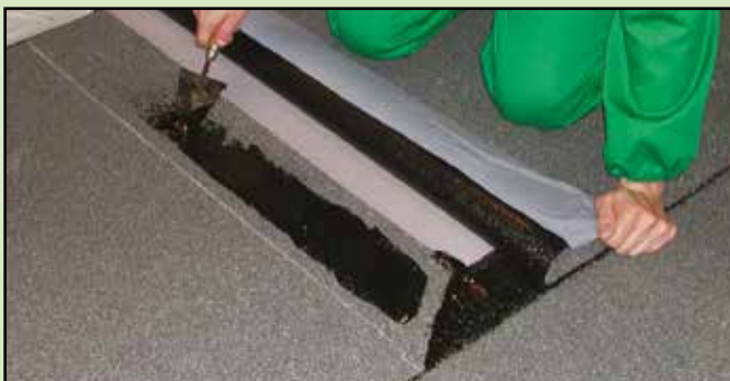
7. Weld the head overlaps with HEADCOLL
