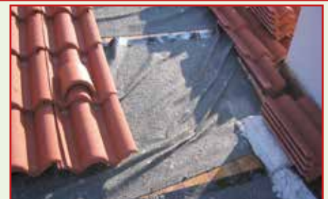
8. Press the whole before applying the tiles
