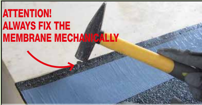
3. Nail the membrane on the strip without adhesive
