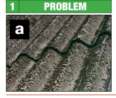
Rendering asbestos cement covering sheets harmless is becoming more and more important for environmental reasons because of the dangers posed by the continuous dispersion of asbestos fibres into the environment.
