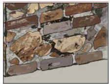
Consolidating old walls while avoiding chemical and physical incompatibility with the wall's materials and salts.
