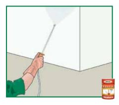
the amount applied is enough to saturate the substrate. Wood, glass and plastic surfaces must be protected during application.
