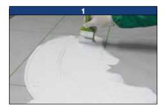
component A and mix thoroughly with a low speed drill to obtain a uniform product. Now gradually add component C while continuing to mix for about 3 minutes, then mix together again until the product is uniform and without lumps. EPOSTOP ABC epoxy cement primer can be applied with a brush, or with a trowel if a thicker application is required (1). Average consumption is 1 kg/m². (For further information about EPOSTOP ABC, refer to the product's technical data sheet).
