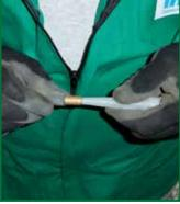
With normal sealant guns the gel is injected starting from the bottom of the hole until the whole cavity is filled leaving the last 2 cm to be filled with quick-setting mortar such as FASTCEM.
