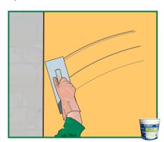
Wall surfaces that have already been painted: remove all traces of flaking paint and any efflorescence. Clean thoroughly, removing dust or dirt and fix the surface with a coat of PRIMER FIX.
