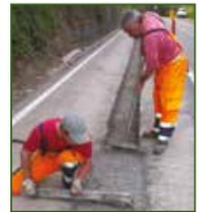
**4.** After the excavation has been filled with the mortar, a strip of the geocomposite membrane, **AUTOTENE ASFALTICO ANTIPUMPING** is to be laid. The membrane is of a breadth of 50 cm (the breadth is that of the scarified zone).
