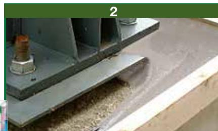
**BETON FLUID RAPID** must be mixed with clean water while maintaining a water/cement ratio lower than 0.40. The mix must be carried out by adding powder to the filler already wet with water (1).
