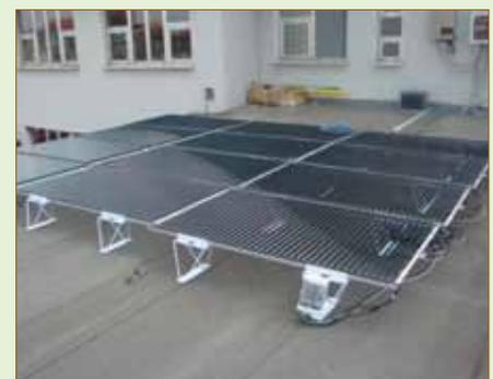
The system dysfunction was due to the bad solar reflectance values of the roof; the subsequent application of **WHITE REFLEX** paint would have demonstrated this hypothesis.
