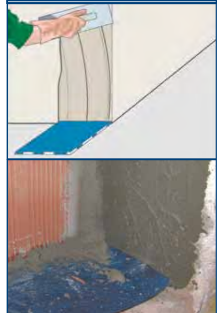
FONOPLAST AND FONOSTRIP KEEP THE WALL SEPARATED RIGHT ALONG THE PERIMETER
