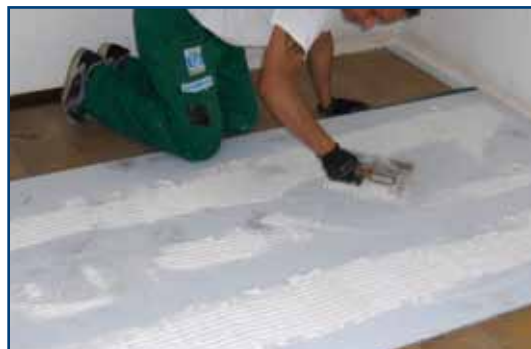
2. Spread the GIPSCOLL glue on the panel
