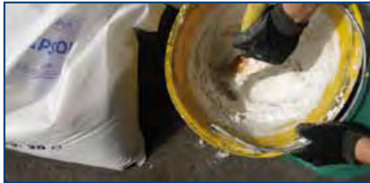
1. Mix the powder glue GIPSCOLL with water.
