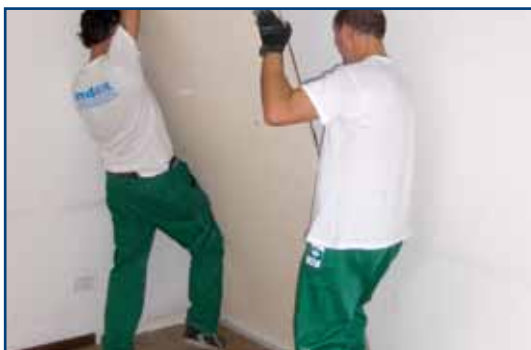
3. Put the panel of TOPSILENTDuogips in position
