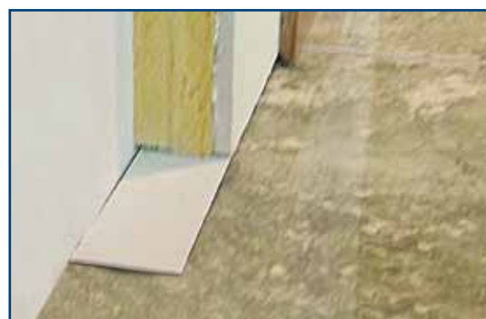
2. Position the sealing strip
