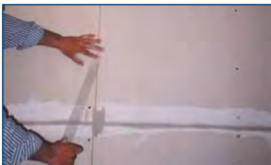
5. Lay and seal of plasterboard
