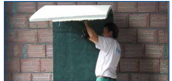
4. Place the panel on the wall.
