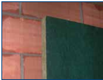
Laying the panels (unpacked version)
