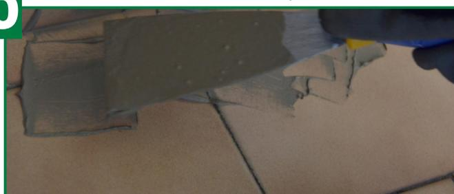
**4** TERMINATE LE FASI PREPARATORIE SI PUÒ PROCEDERE ALLA STESURA DI HYDROSEAL. LA STESURA DEL PRODOTTO PUÒ ESSERE ESEGUITA IN DUE MODI: CON PENNELLO O IRRORATORI A BASSA PRESSIONE, IN UNA SOLA MANO, INSISTENDO PARTICOLARMENTE NELLE FUGHE E NELLE ZONE PIÙ ASSORBENTI IN MODO DA PERMETTERE ALLA SOLUZIONE IMPERMEABILIZZANTE DI IMPREGNARE OGNI POROSITÀ.
